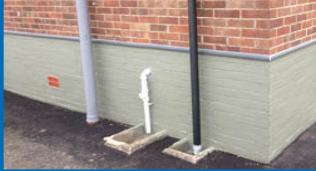
Non-Return Valve for smaller waste pipes
